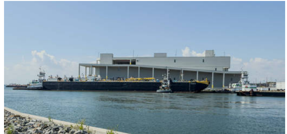
Fig. 16 Two-story logistics facility on Gowanus with fuel barges in the foreground. Photo: Tom Fox.
