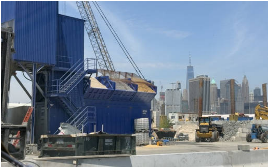
Fig. 32 Prefabricating concrete structures. Photo: Tom Fox.
