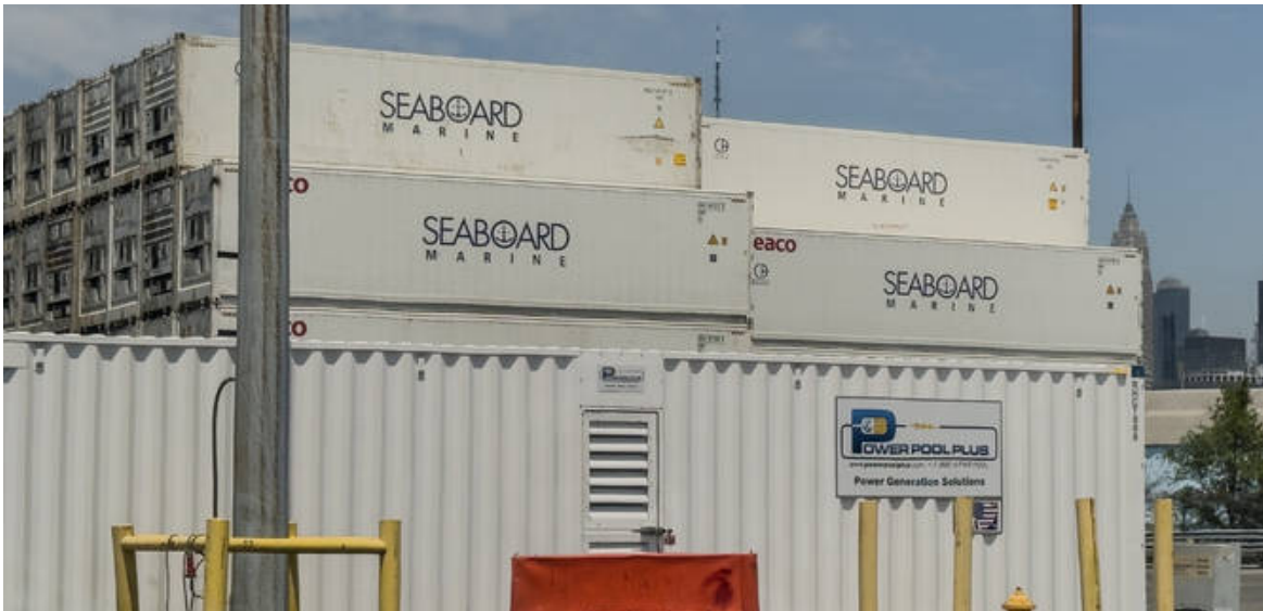
Fig. 23 Seaboard refrigerated containers. Photo: Tom Fox.
